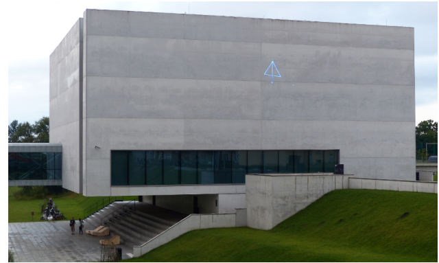
Figure 6. Building with overhang unsupported on pillars, requiring adjustment for surface area of internal walls in object EGB_BlokBudynku
