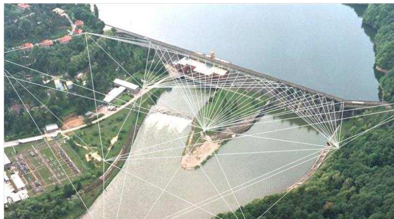
Fig.1. Rożnów dam on the Dunajec river with inscribed trigonometric network, geometry affixed for horizontal shift study
