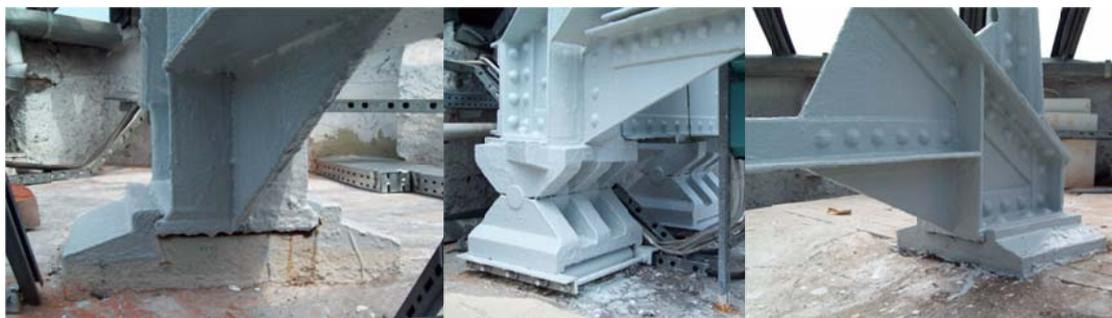
**Fig. 14.** Movable mount of the construction on bearings C, D and E
