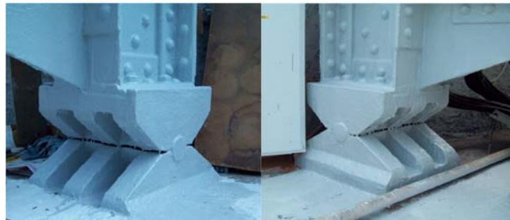
**Fig. 13.** Jointed mount of the construction on bearings A and B
