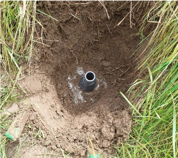
Figure 8. Placing the conical head on a benchmark approximately 63 mm in diameter with the axis vertical, before setting up the GNSS antenna precision forced centering device
