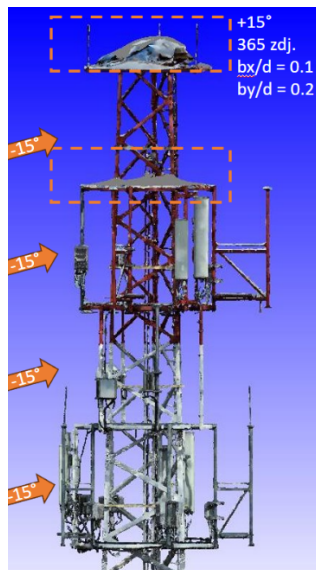
Figure 5: Geometric artifacts in areas occluded by objects on the maintenance platform and fixed camera pitch angle (orange boxes). Orange arrows — approximate elevation and camera pitch of “orbits”
